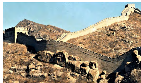
The Great Wall of China
